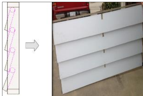
Figure 6 Louver style panels which can only open in one direction
