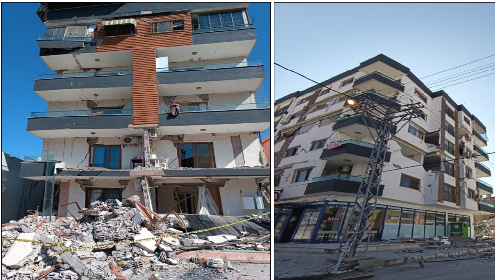
Figure 1 Irreparable Damage to One- and Two-Year-Old Buildings During the Kahramanmaraş Earthquake
